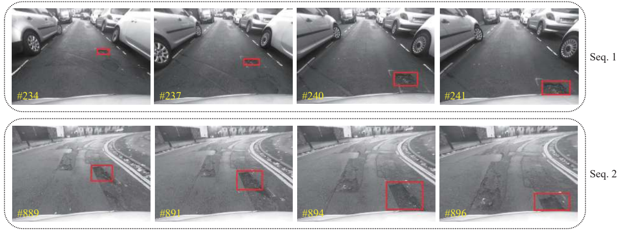
Fig. 4. Pothole tracking results. The (same) potholes in different video frames are tracked with scale-adaptive bounding boxes.
